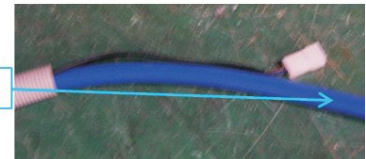
Connecting to air breaker
