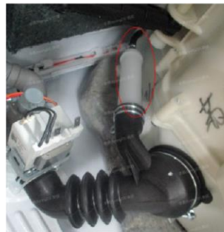
Fig.7 Whether the air pipe is damaged
