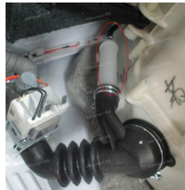
Fig.7 Whether the air pipe is damaged
